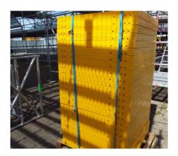
Place the legs neatly in the decking leg pallet provided in stacks of 56 as per image.
